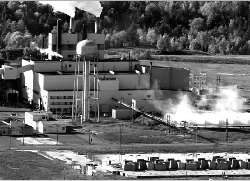
The 40-megawatt plant in White Pine will be converted from coal to biomass using the existing infrastructure. The engineering prefesability study is underway and environmental permitting will be submitted in early January 2010.
